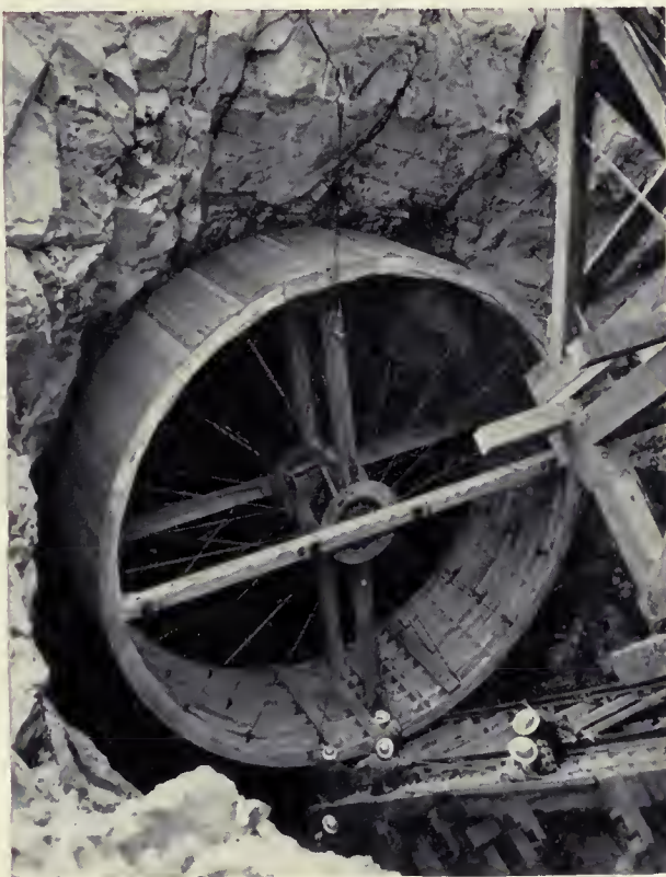
FERRIS-WHEEL form, man-made "geysers," and follower gates. Photos by A. E. McCloud and A. G. Rainwater, of Region 1.
